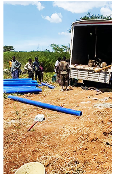
Onsite at a bore drilling site in Tanzania.
